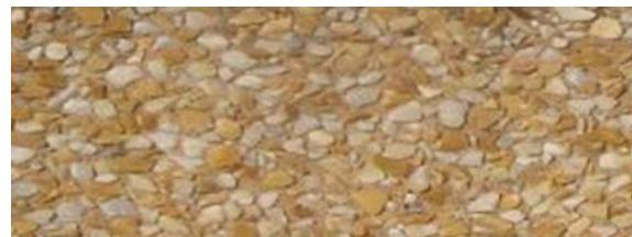
The washing depth and granulometry values recommended are approximate, as they depend on many factors: the correct and uniform application of the product, the type and quantity of cement, the water / cement ratio, granulometry mix size and fineness amount as well as time and temperature of the curing process.
